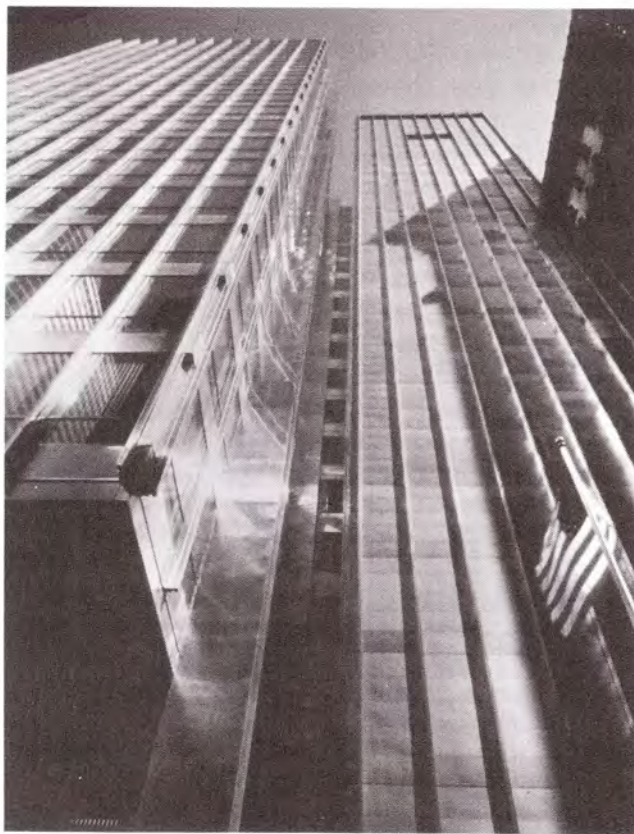
Chicago's stainless-steel-clad Inland Steel Building (1955-57), by international style architects Skidmore, Owings and Merrill, paved the way for new cladding materials. (Photo by Jon Miller/Hedrich-Blessing. Courtesy of Skidmore, Owings and Merrill)
