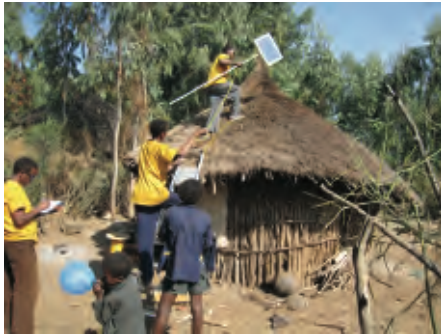
Solar technicians installing a hut
