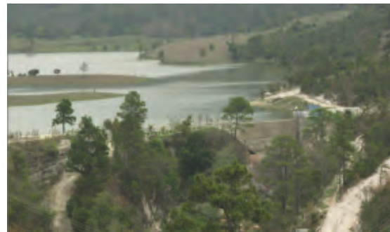
LaEsparanza hydroelectric plant, Nicaragua E+Co supported growth from 485kW to 13MW
