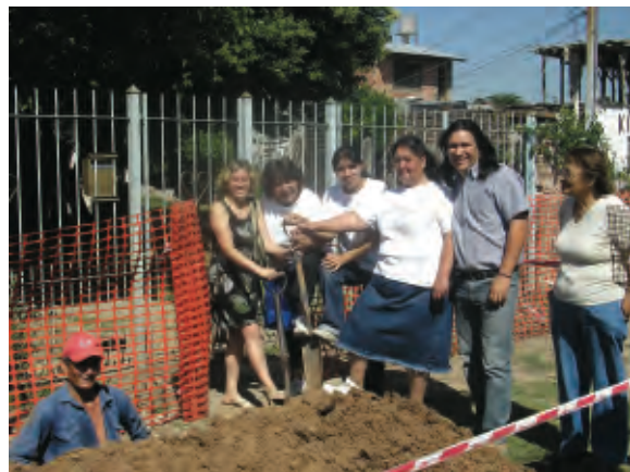
Figure 6 Crew working outside Buenos Aires
